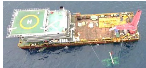
Offshore Installation of Subsea Manifolds
