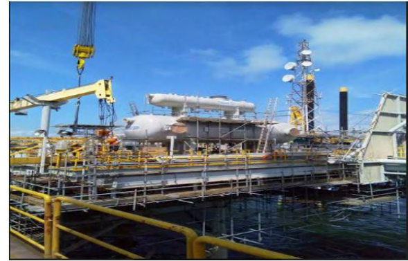
COMPLETED INSTALLATION OF HP & TEST SEPARATOR ON MEJI RP
