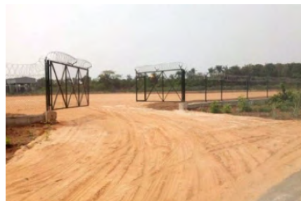
SITE PREPARATION FOR COMPRESSOR STATION
