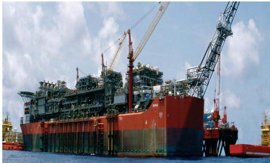
Bonga Main Life Extension project
