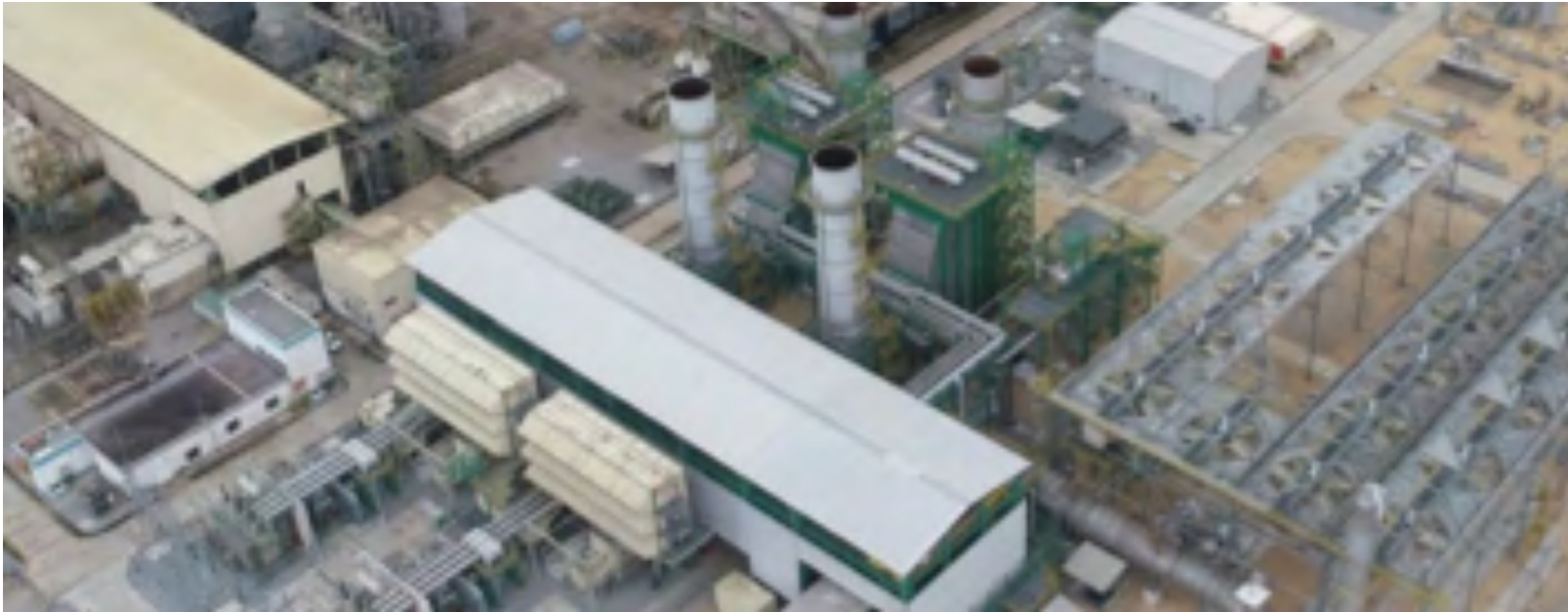
Okpai IPP Phase 2 Project
