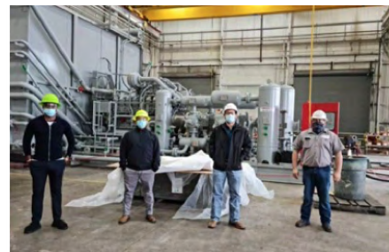
FAT OF AG COMPRESSOR PACKAGE
