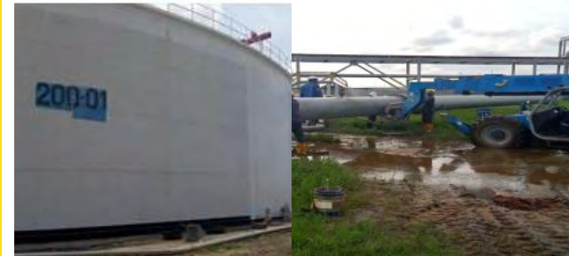
Coating of stained sections on Tank 1 shell
