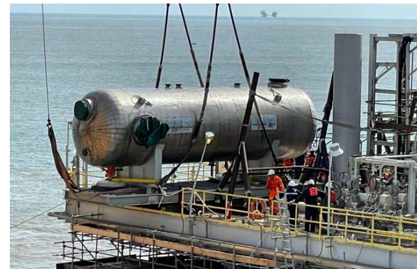
Completed Slug Catcher Installation
