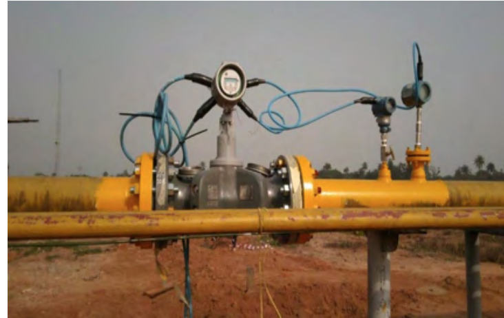
COMMISSIONED GAS IN-PLANT METER
