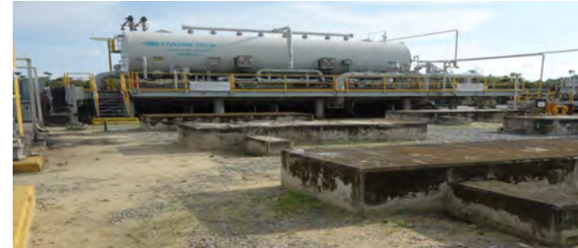
Installed Envirocell#1 and completed foundations for pipeline pumps
