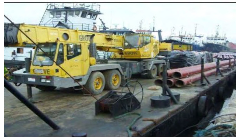
Community Provided Crane
