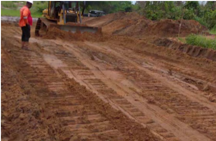
EXCAVATION OF ACCESS ROAD TO RECEIVE FILL MATERIAL
