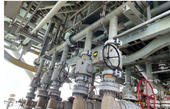
Completed NWP Manifold Modification
