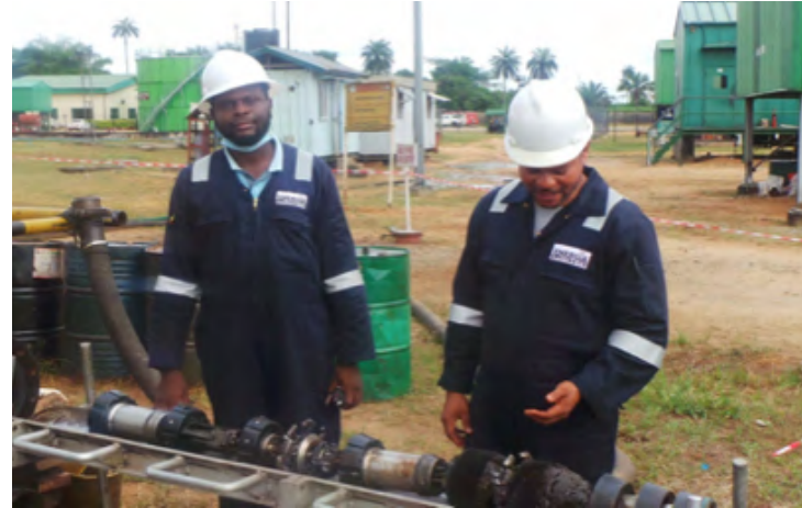
INSPECTION OF PIG CONDITION BY ENERZIA PERSONNEL
