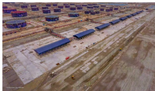
PRODUCT TANKS WITH LOADING GANTRY
