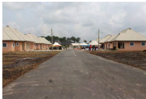
EBENDO HOUSING ESTATE & INTERNAL ROADS
