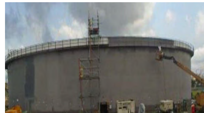
Blasting and painting of Tank 2 external shell
