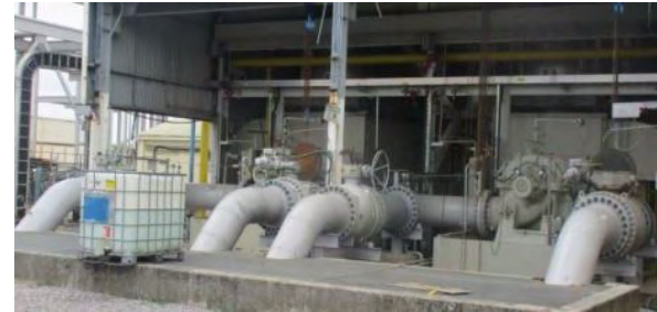
Pump House B with 2 Turbine-Driven Pumps Installed
