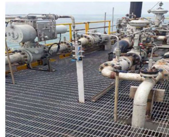
GRATINGS & HANDRAILS INSTALLED AT THE LAST DECK OF THE MODULE
