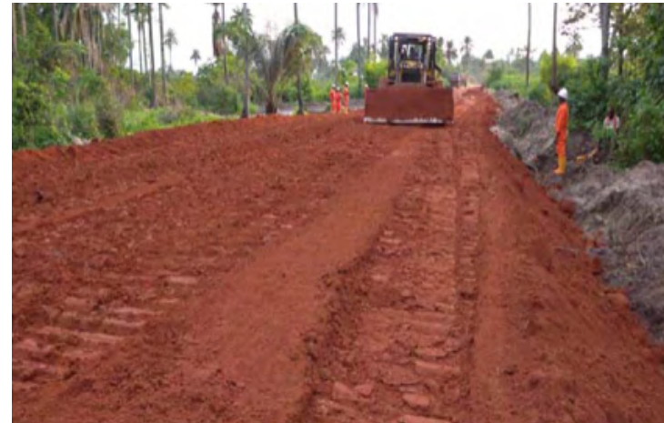
LATERITE FILLING AND COMPACTION OF THE ACCESS ROAD
