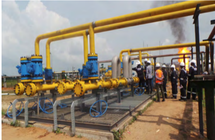
GAS CUSTODY TRANSFER METER
