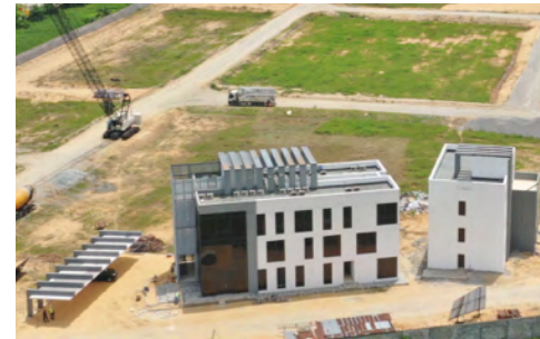
ADMINISTRATION AND TERMINAL OPERATOR BUILDINGS
