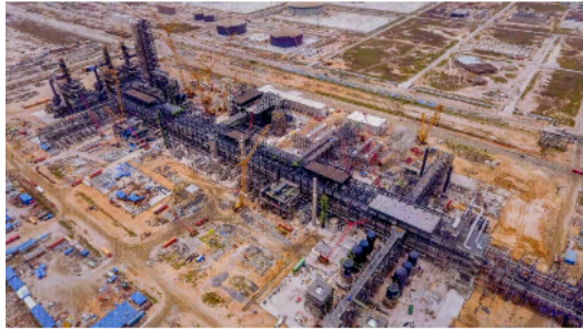
CRUDE DISTILLATION UNIT
