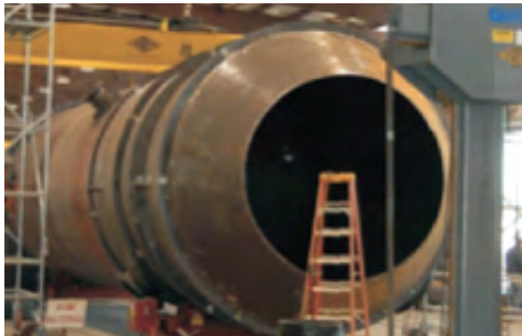
CRUDE DISTILLATION UNIT
